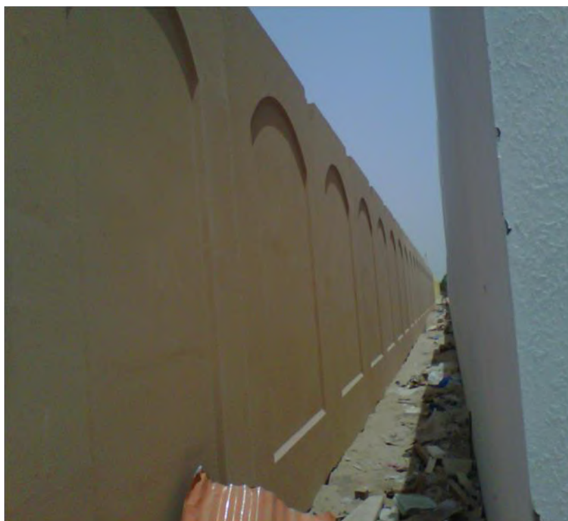
Figure Seven. Space between property boundaries creates unofficial footpaths in Abu Dhabi
