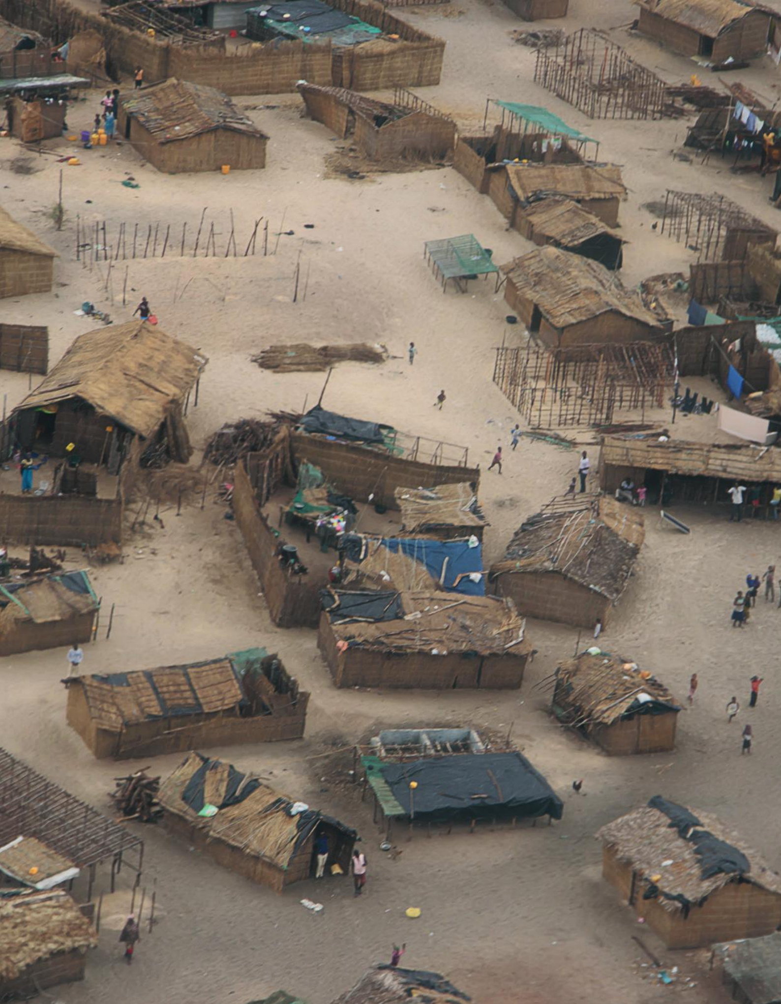
Aftermath of Cyclones Idai and Kenneth in Mozambique in 2019
